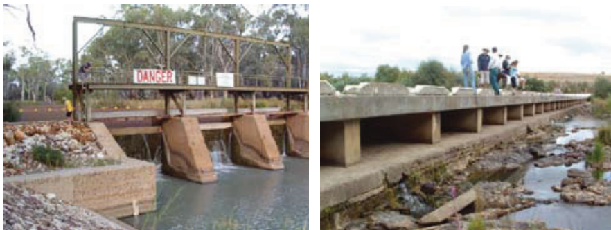
At left – in-stream weir regulating flows. At right – road crossing impacting on flow patterns. Photographs: Bill Phillips
